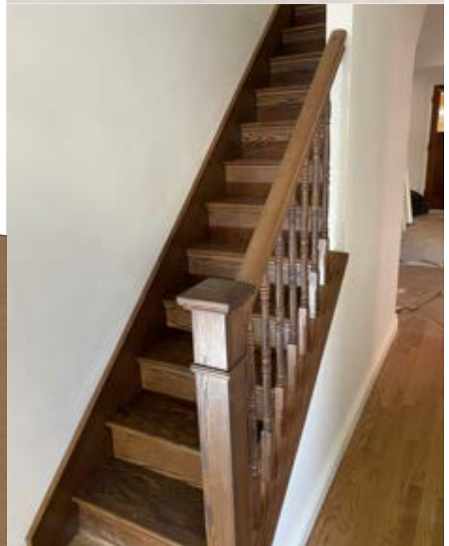
STAIR RECAP & NEW RAILINGS
