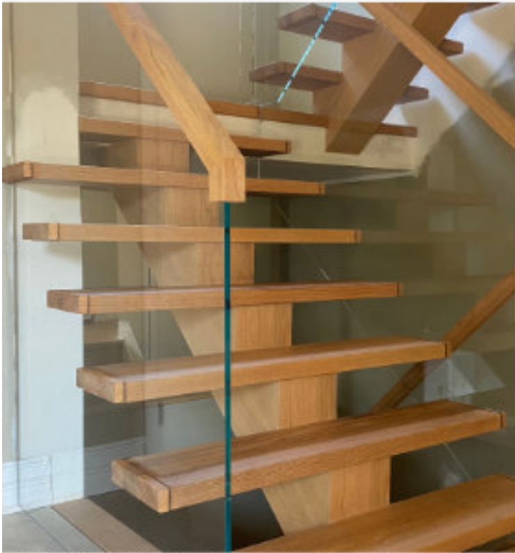
NEW STAIRS & RAILINGS
