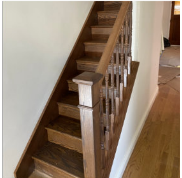
STAIR RECAP & NEW RAILINGS
